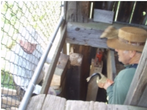
The deteriorated sill plate can be seen just below the raw wood of the replacement sill, sawn to size by the mill crew last year.
