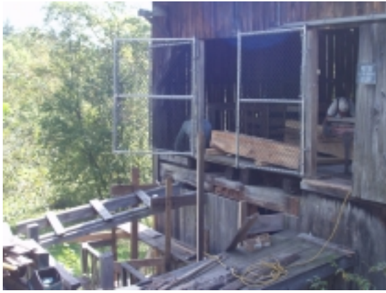
The deteriorated sill plate can be seen just below the raw wood of the replacement sill, sawn to size by the mill crew last year.
